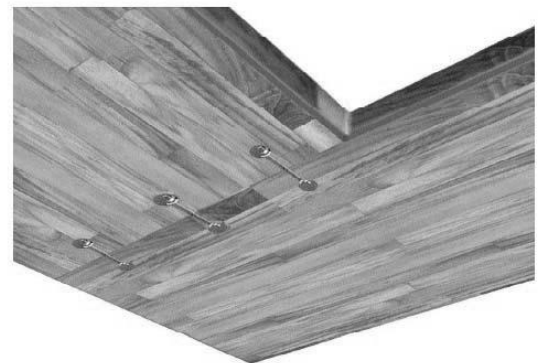
Fig. 9 Completed butt joint (underside)
