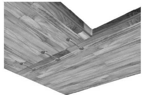
Fig. 9 Completed butt joint (underside)
